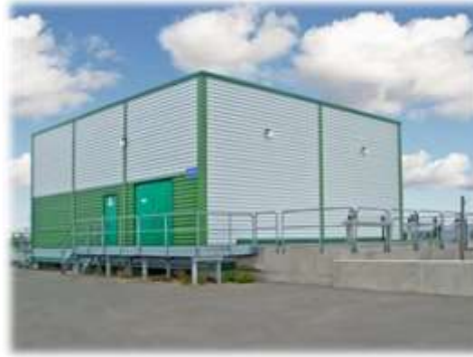
South-West WWTP, St. Petersburg Russia - 330,000 m 3 /day
