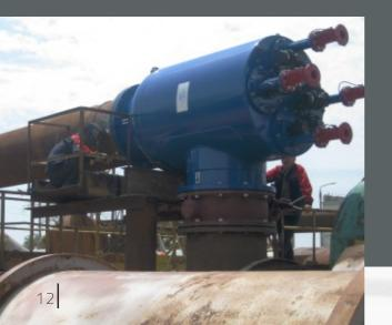
**Brush - MGB** Electric multi-screen brush scanner self-cleaning screen filter for very high flows. Filtration range: 2000-3000 micron In/out Diameter: 16" – 54"
