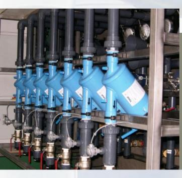
**Industrial Machine Protection** In-out diameters: F-100 – from 1.5" - 10" F-200 – from 1.5" - 10" F-300 – from 2" - 6" F-400 – from 1.5" - 10"
