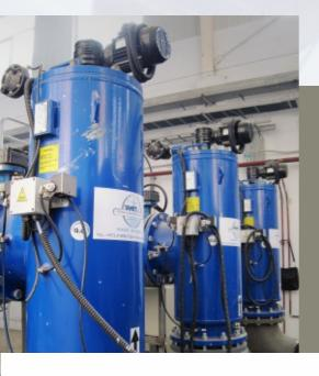
**AF-700/7500** Electric brush scanner self-cleaning screen filter. Filtration range: 200-3000 micron In/out Diameter: 4″ – 16″
