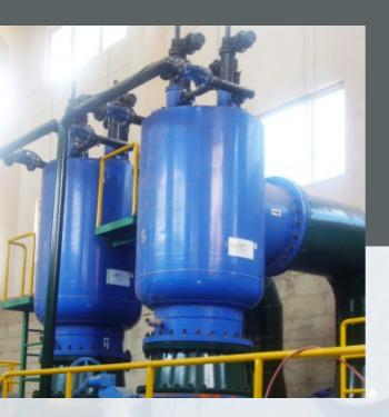
**Electric - MGE** Electric multi-screen suction scanner self-cleaning screen filter for very high flows. Filtration range: 10-3000 micron In/out Diameter: 16" – 54"
